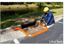
**Berms:** Manufactured berms can be used if grading is adequate and there are relatively smooth drainage surfaces, They can encircle a storm drain, allowing water to pond for later collection or diversion to the sanitary sewer.
