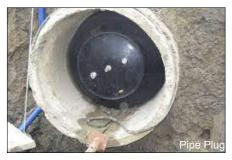
**Inflatable Pipe Plug:** The plugs are inserted into a storm drain pipe and inflated for a tight fit to prevent washwater from entering the pipe. Washwater is collected in the storm drain sump and then pumped to a holding tank or sanitary sewer.
