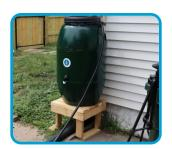
Level the area where the stand and barrel will be located. Place barrel on the stand beneath the downspout. Mark where to cut the downspout for the diverter or downspout elbow.
