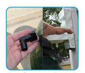
For overflow, install a diverter on the downspout that can be closed when the barrel is full. Or attach an elbow to the downspout and install an overflow fitting on the barrel to connect a hose to redirect overflow.
