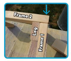
Screw the free end of each frame piece into the leg end of the next frame piece.
