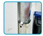
Install diverter (shown) by putting a sheet metal screws through the tabs and downspout, or downspout elbow with sheet metal screws and screwdriver.
