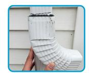
Cut the downspout with a reciprocating saw like a Sawzall or a hack saw. Make sure the cut is straight.
