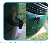
Drill a hole near the bottom for the spigot. Drill a hole near the top if needed for an overflow fitting (diverter not used).
